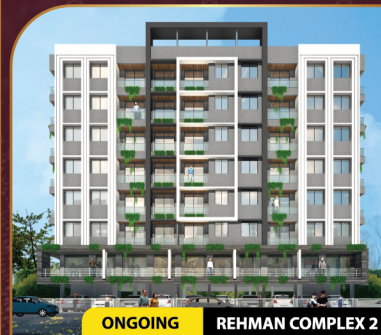
ONGOING REHMAN COMPLEX 2
